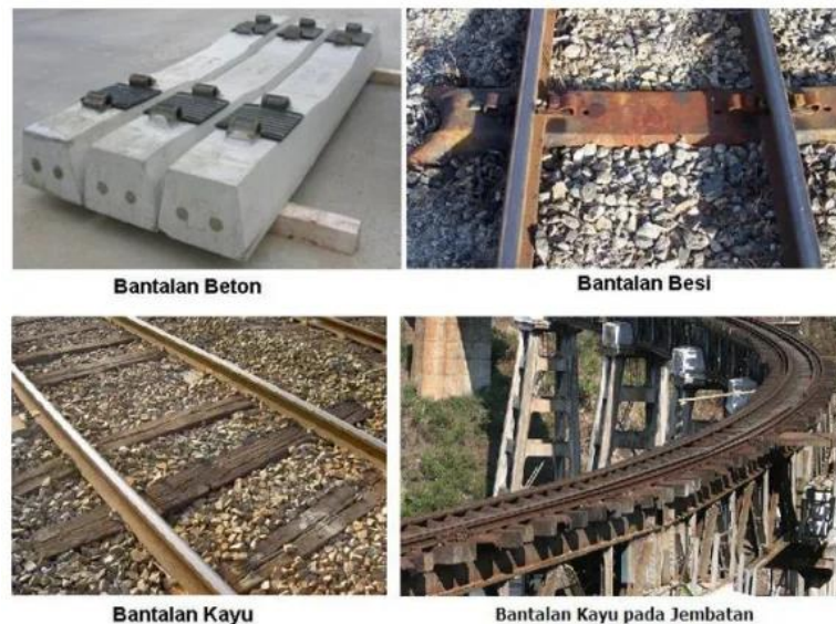
Figure 2. Different kinds of railroad bearing
