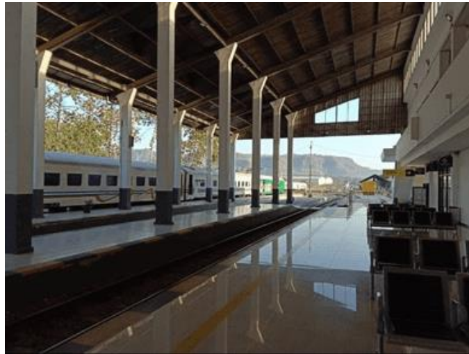
Figure 3. Waiting Room at Station
